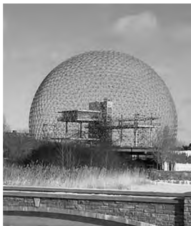
Figure 2.2 With his geodesic domes, R. Buckminster Fuller provided the architectonic inspiration for the naming of the fullerenes. The US pavilion for the Montréal EXPO76 is just one example (© Montréalais).
